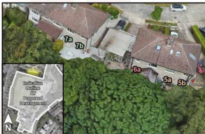
Fig. 5.5: Affected windows Norwood Park.
